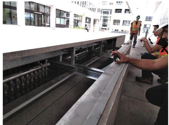
The Calgary-based company’s PEX snow and ice melt system eliminates the need for those other methods, helps to preserve the manufactured stone finish without abrasion caused by shovels or chemical attack from salt, and ensures pedestrians can safely and comfortably enjoy the space and use the stairs at any time of day or night in the wintertime.
